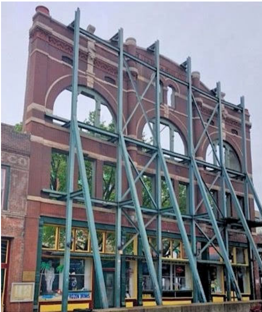
Silky O'Sullivan's patio (formerly Gallina Exchange Building), built 1891.
