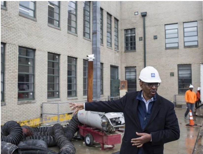
Jimmie Tucker guides a tour of the renovation to the Universal Life Insurance building March 16, 2018. (Photo: Brad Vest / The Commercial Appeal)
